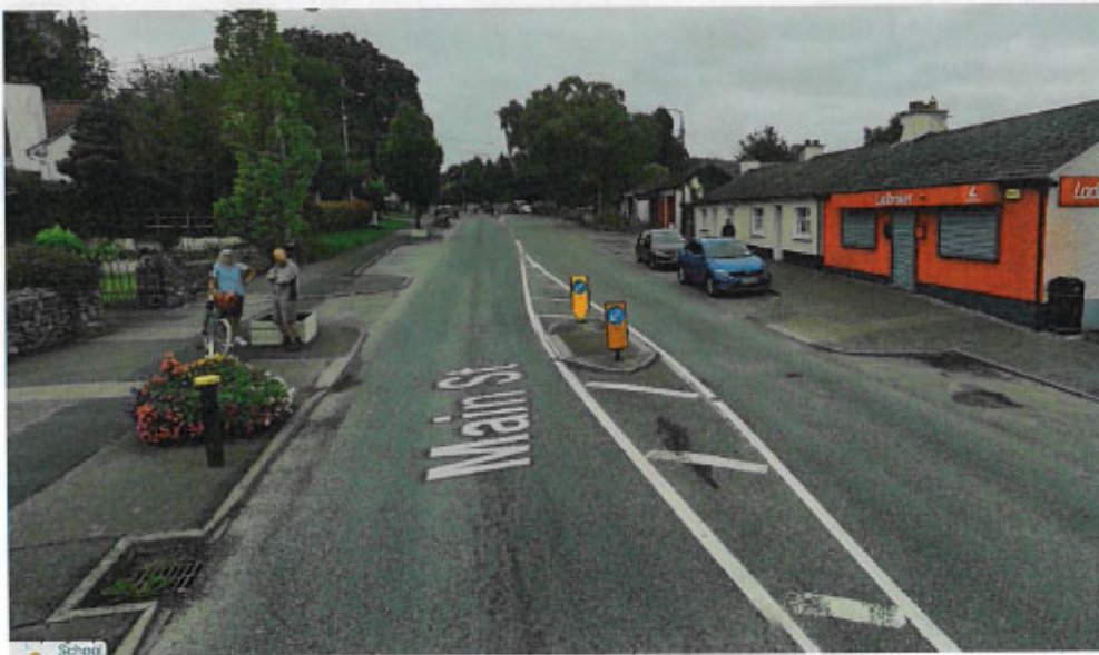
Adjacent The Old House Public House - Proposed development shows this refuge being removed without substitute traffic calming.
