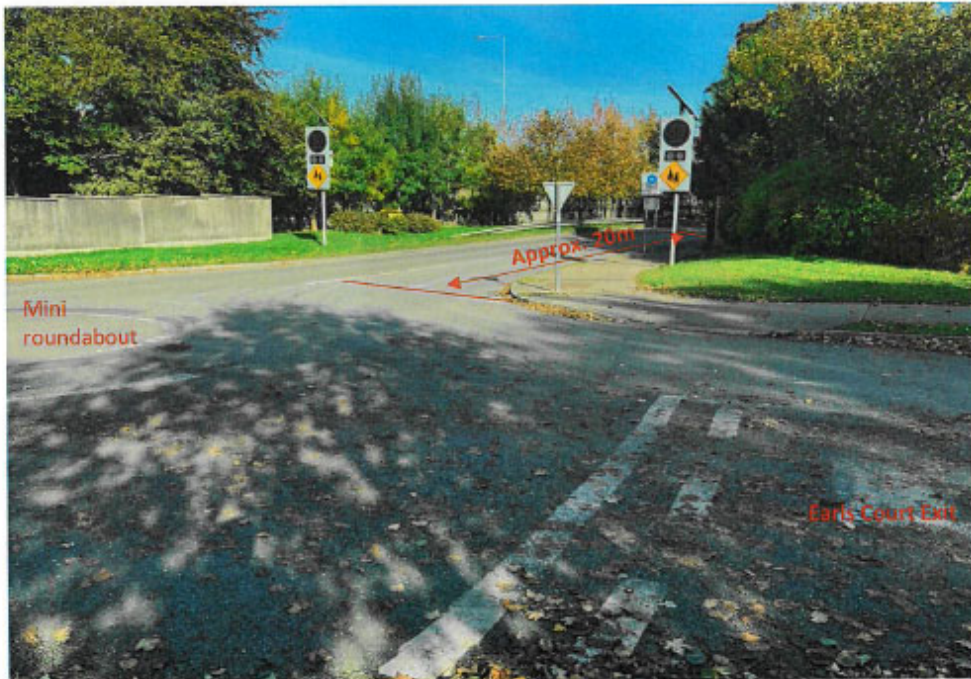
Showing current extremely limited sightline east from exit of Earls Court.
