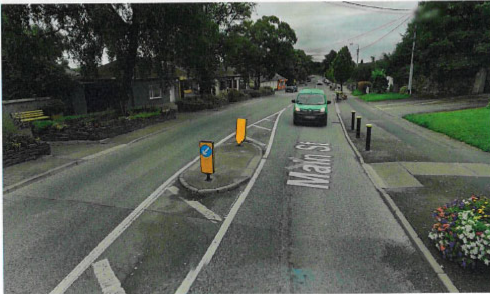
Adjacent St. Johns Church - Proposed development shows this refuge being removed without substitute traffic calming.
