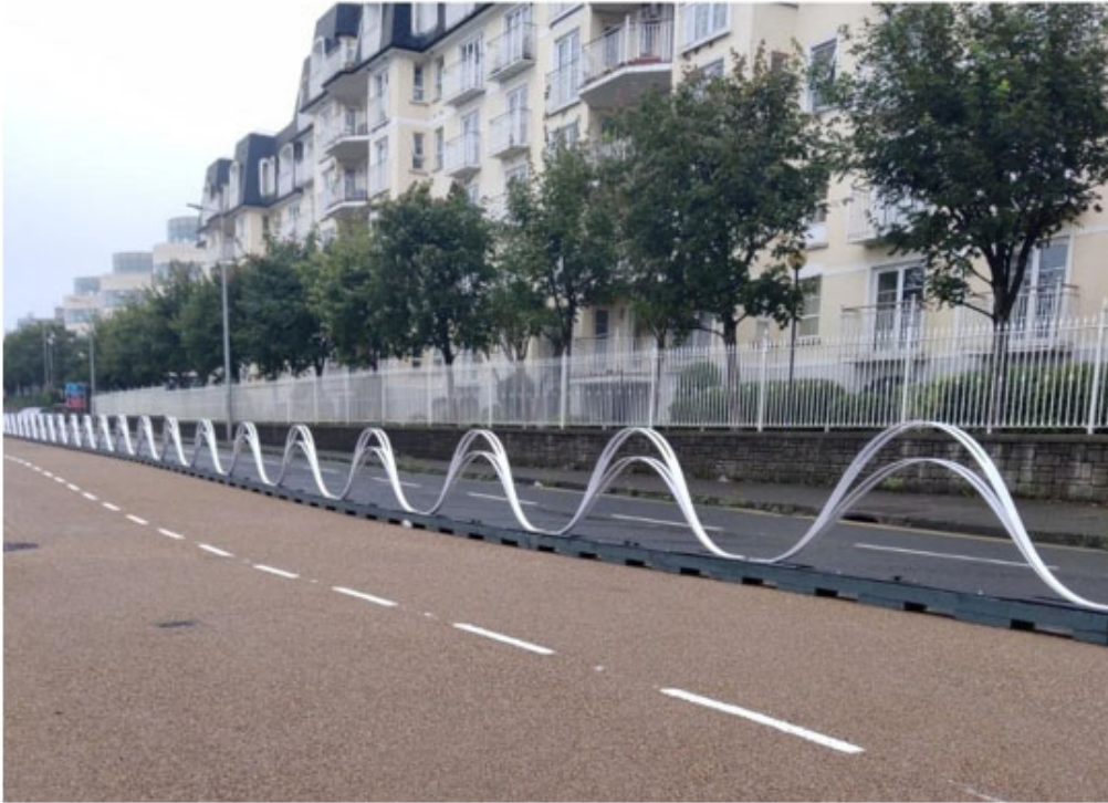
Figure 1: Example of cycle lane and carriageway divider from DLR
